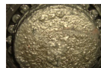
Bearing Condition with Previous Grease
